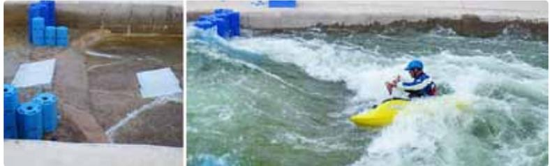
The course, which opened in 2010, has shallow and surging water. They needed a safe feature former on the floor that the rival obstacle system, already installed, couldn't offer. Our wave forming wedges provided smooth flow transitions for green surf waves in this low flow course.
