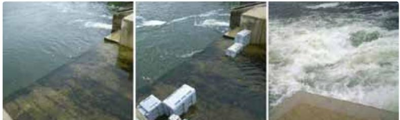
An experimental installation to demonstrate the ease of installing RapidBlocs during weir refurbishment; making a recreational feature from an otherwise single purpose structure.
